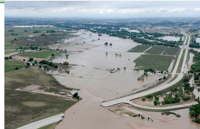
Sept. 16, 2013: U.S. Highway 34 in Greeley is breached by the South Platte River in flood stage. (Credit: US Environmental Protection Agency)
